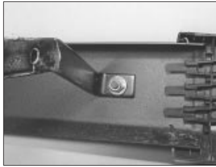
16.19a Courier rear bumper removed, showing mounting bracket retaining nut and end moulding clips . . .
